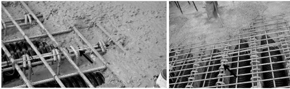
Figure 2. Embedding in concrete of long-gauge sensors (sensor indicated with arrow).
