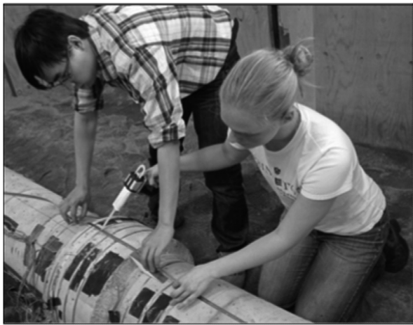
Figure 8. Gluing of sensors, detail at joint (second test).
