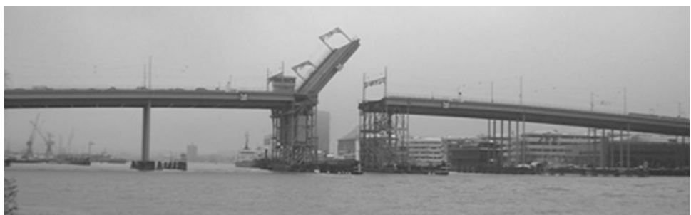
Fig. 1 Side view of the Götaälv Bridge during bridge opening
