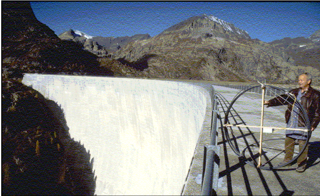
Figure 7.3.2: Emosson dam and Long Sensor on transporting spool
