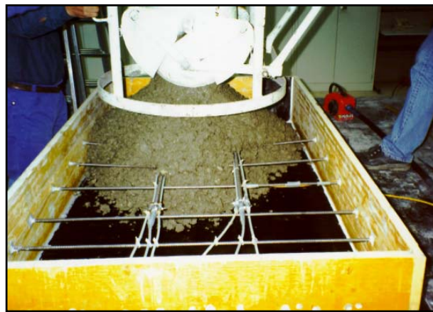
Figure 6.3.3.3: Pouring of concrete slab with thermocouple, Stiff and Standard Sensor
