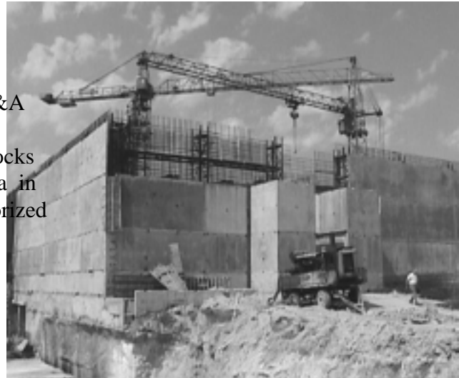
Figure 4. High-security fissile-material storage facility under construction in Ozersk
