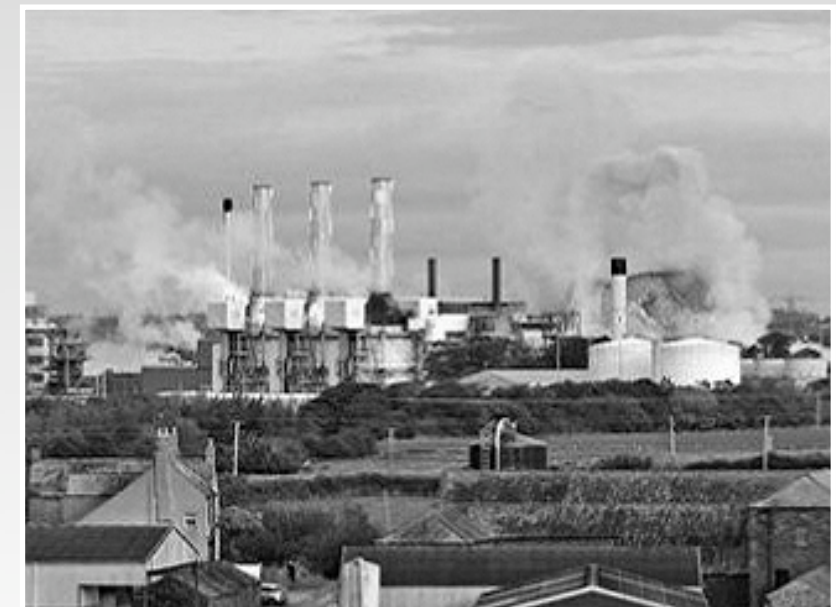
Demolition of Calder Hall (A) Towers September 29, 2007
