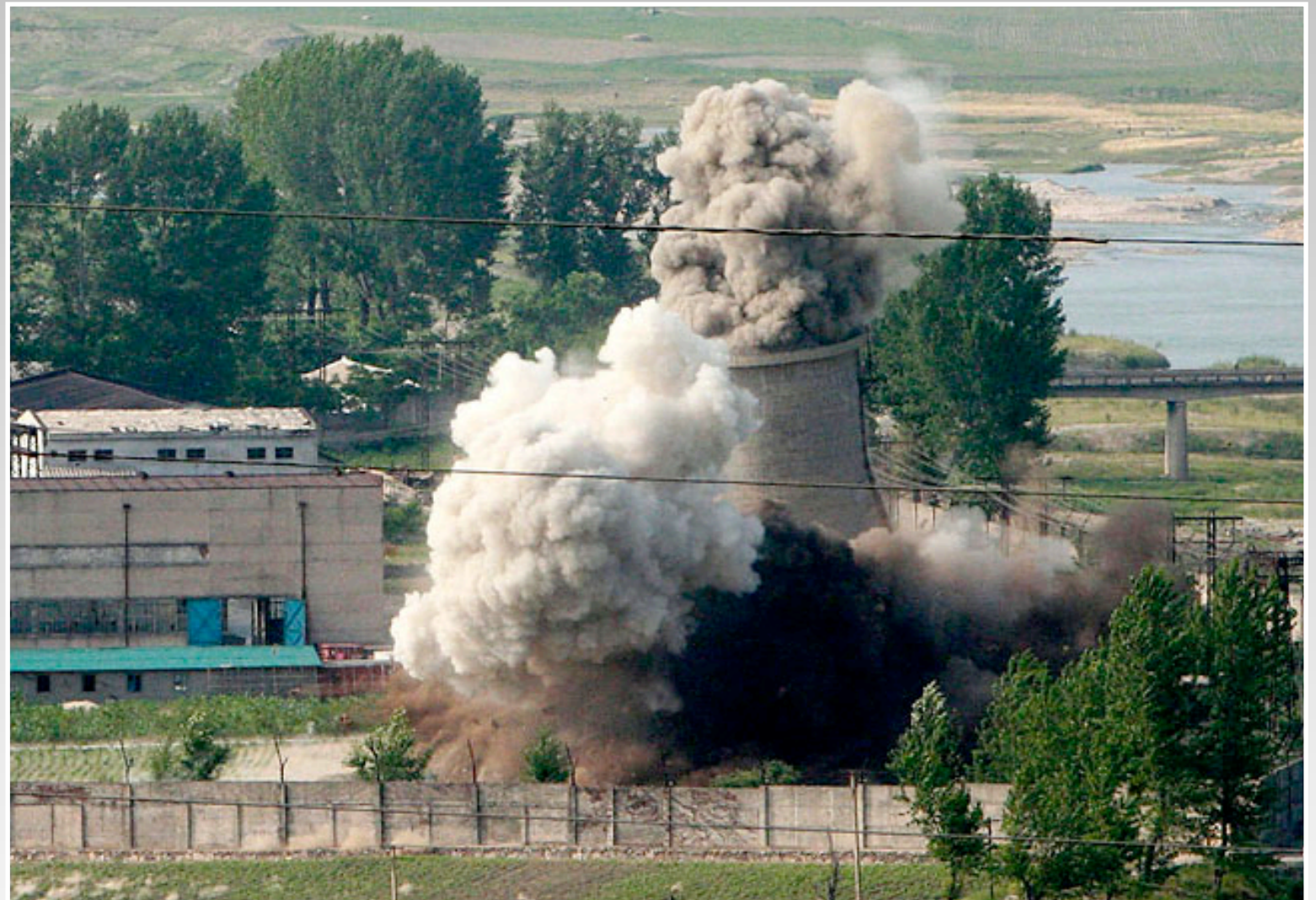
Demolition of cooling tower, June 26, 2008
