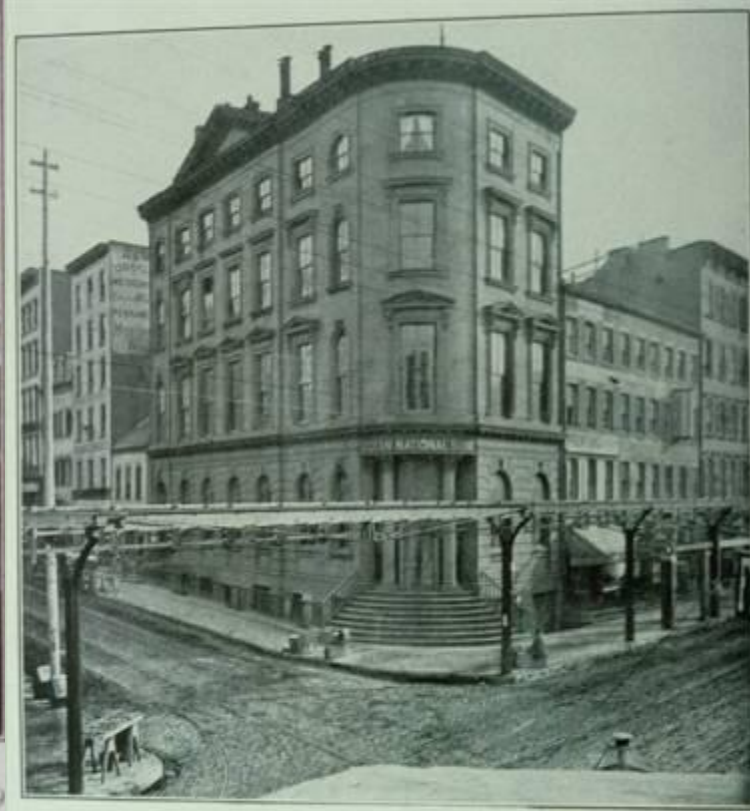
GREENWICH STREET, LOOKING SOUTHEAST FROM THE CORNER OF FULTON STREET, 1869 Showing the first elevated railroad, erected 1868-69 on the easterly curb line of Greenwich Street in front of the Ocean National Bank, and operated by cable.
