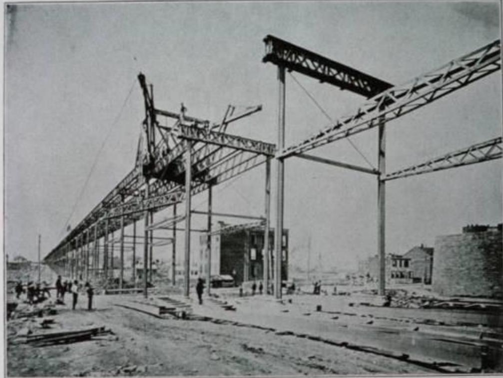
STRUCTURE OF THE METROPOLITAN ELEVATED RAILWAY COMPANY (SIXTH AVENUE LINE) BEING ERRECTED ON NINTH AVENUE (COLUMBUS AVENUE) IN 1878-79
