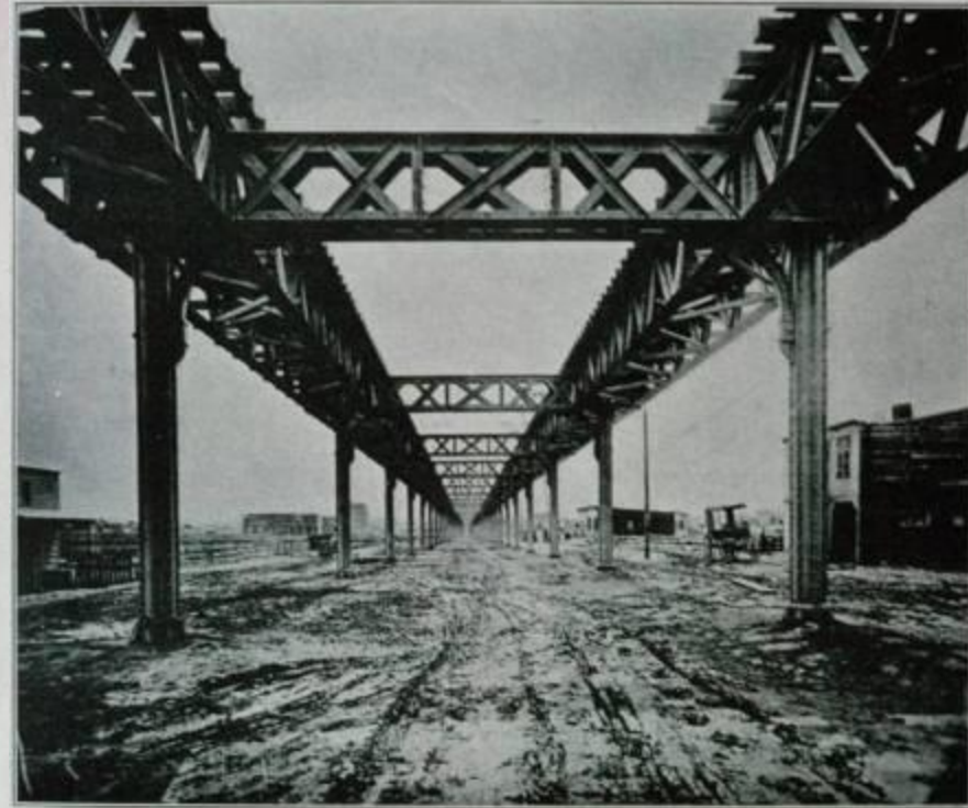
TWO-TRACK JOINT STRUCTURE OF THE NEW YORK ELEVATED RAILROAD (NINTH AVENUE LINE) AND THE METROPOLITAN ELEVATED RAILWAY (SIXTH AVENUE LINE) ON NINTH AVENUE (COLUMBUS AVENUE), LOOKING SOUTH FROM WEST 83RD STREET, IN 1878-79
