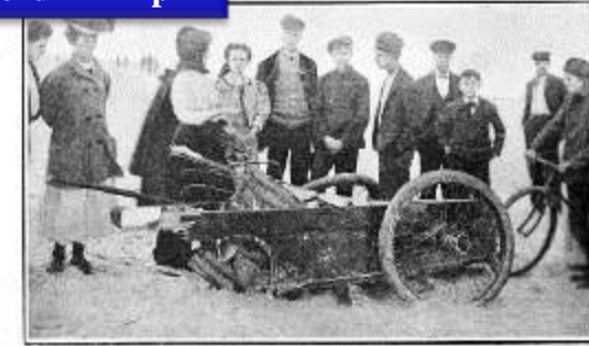
Part of the Body of Haver After the Accident. THE ACCIDENT TO THE STANLEY STEAM RACER CAN AT BRIDGE BRIDGE.
