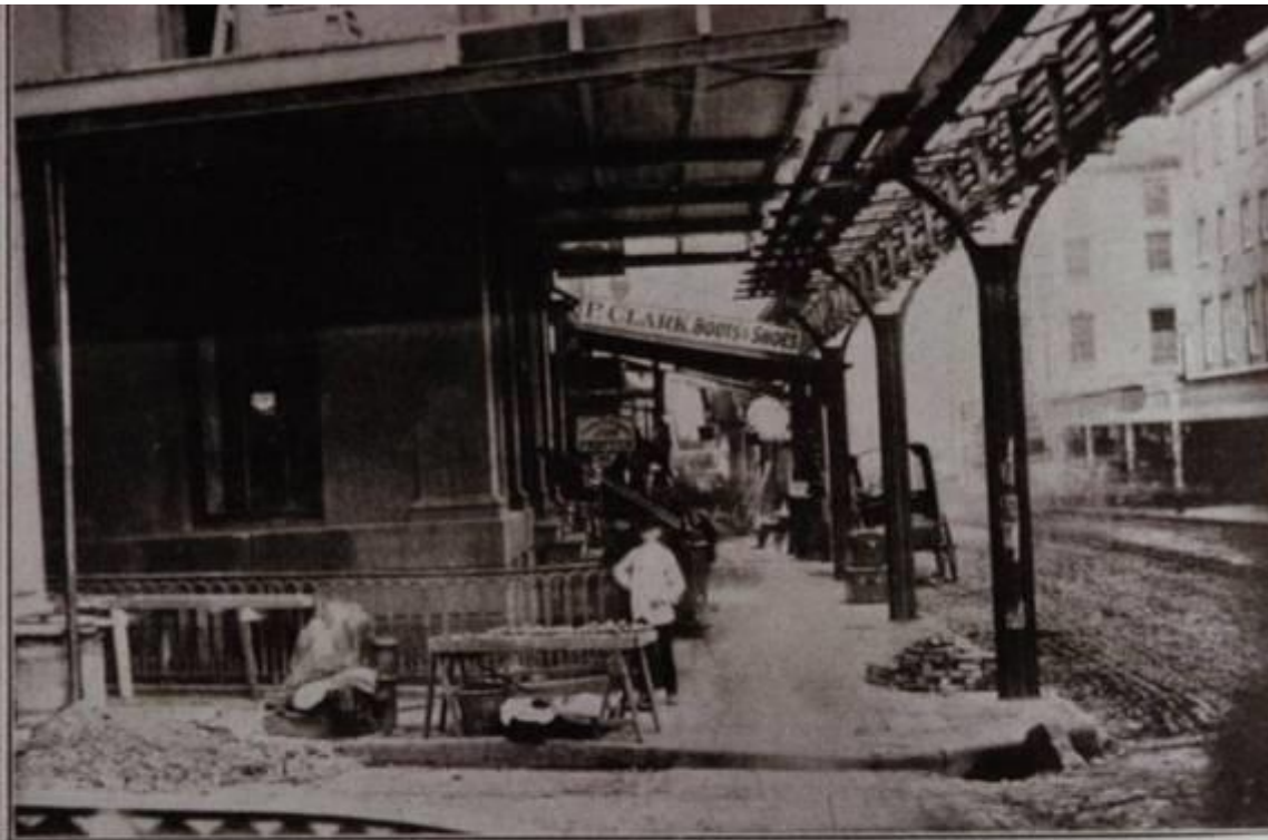
GREENWICH STREET LOOKING SOUTHEAST FROM DEY STREET, 1868-69 Showing the elevated structure on the east curb line of Greenwich Street, built in 1868-69, cable used for train operation, showing the first south station at Dey and Greenwich Streets in course of construction.
