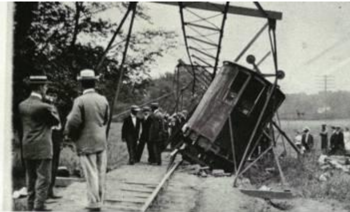
End of a bright dream: a wrecking crew props up the toppled Pelham Bay monorail car. Note the single rail on the ground.
