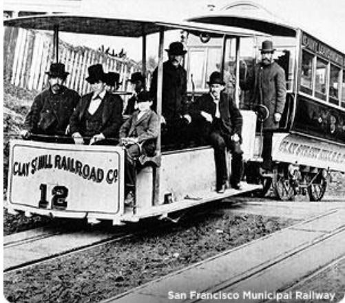
Beginning in 1873: San Francisco
