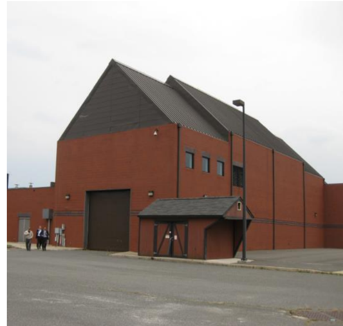
Unique facilities – McAfee Center - entrance to large vehicle bay
