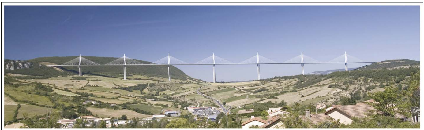
Figure 1. Norman Foster’s viaduct across the Millau Valley in the Languedoc region of France.
