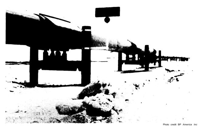
Mile Zero, Start of the Trans Alaska Pipeline at Prudhoe Bay. The elevated pipeline rests on structures called vertical support members (VSMs).
