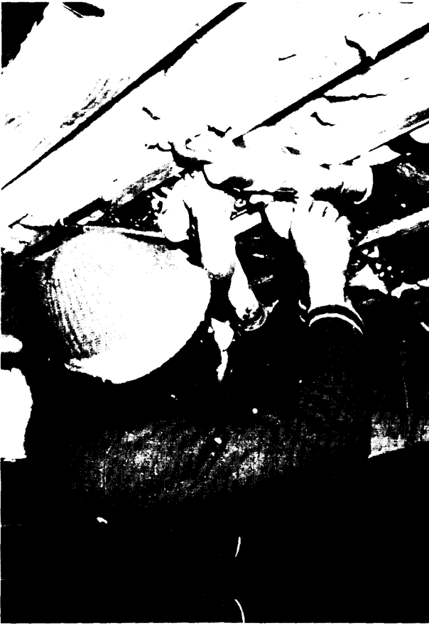
Photo credit: Dr. J. Hill, U.S. Department of Commerce, National Institute of Standards and Technology, Building Environment Division
