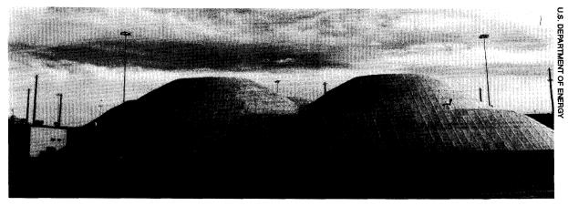
Explosion-resistant warhead disassembly cells at Pantex (Gravel Gerties).
