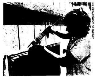
Caulking gaps around windows and doors can reduce infiltration, and thereby reduce energy use for space heating and cooling.
