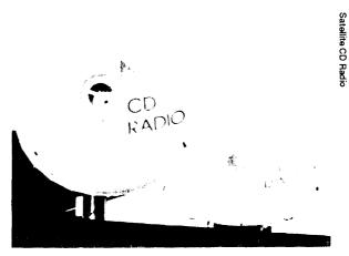
Satellite dishes such as these will beam digital quality radio programming up to satellites that will then retransmit it across the country.
