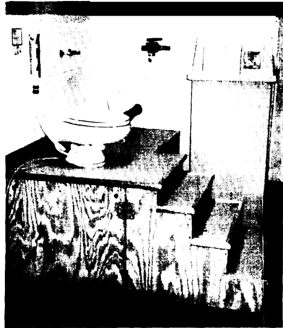
FIGURE 5-1: Cowater Sanitation System Showing Water Storage Tank and Toilet Installed Over Indoor Holding Tank
