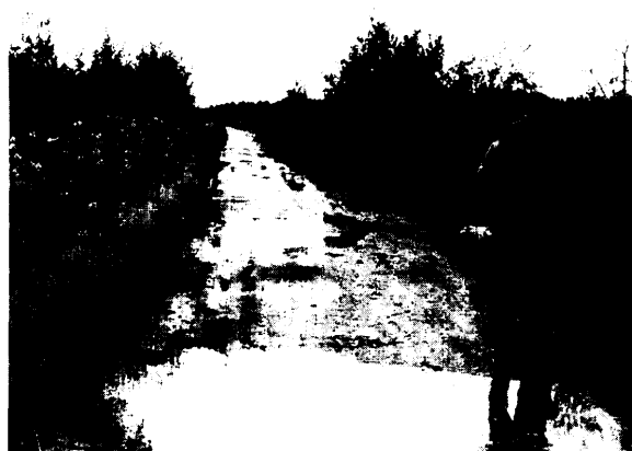
The inadequate condition of roads in some villages often results in spillage of human waste during its transportation to disposal sites
