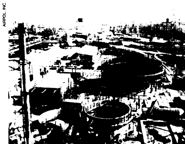
The early stages of assembly at the Skawina plant site. In the background is the thickener with preassembled sections of the absorber vessel in the foreground. The absorber vessel sections are ready to be placed in position
