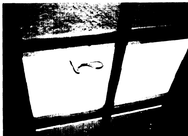
The imitation snake represents a “low-tech” solution to the problem of damage from bird droppings.
