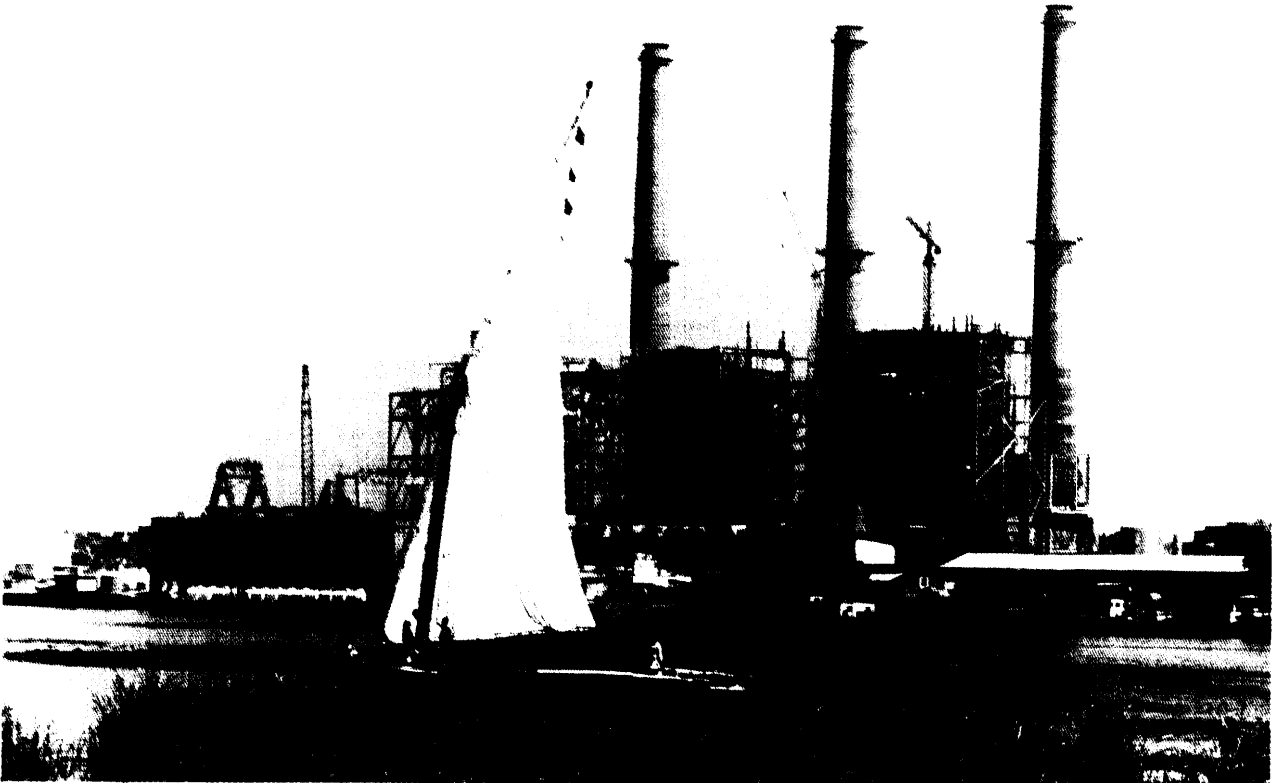
Photo credit Bechtel Power Corp
