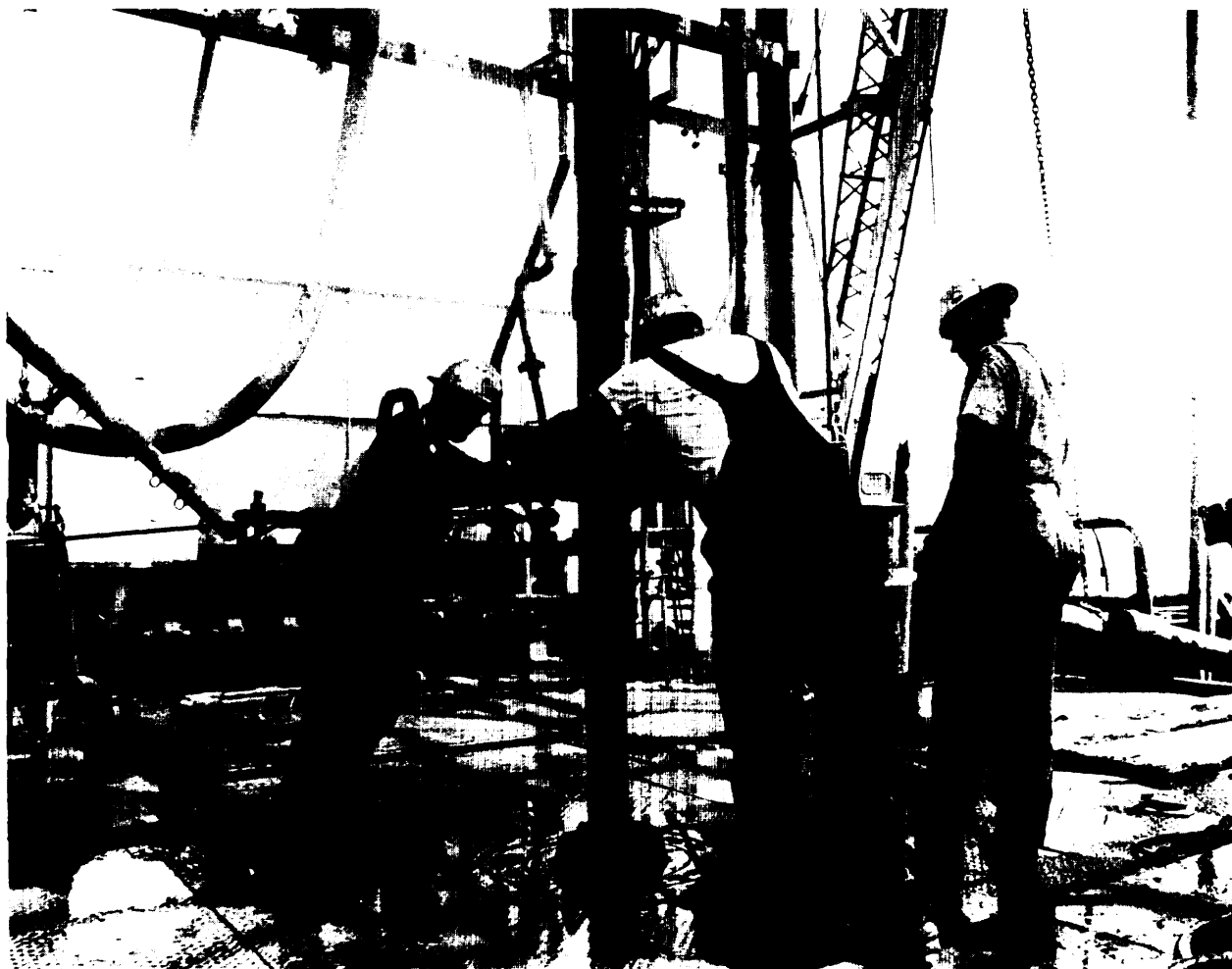
Figure IV-12. Drilling crews work with the drill string at an offshore well similar to those which will be put down in the Mid-Atlantic.
