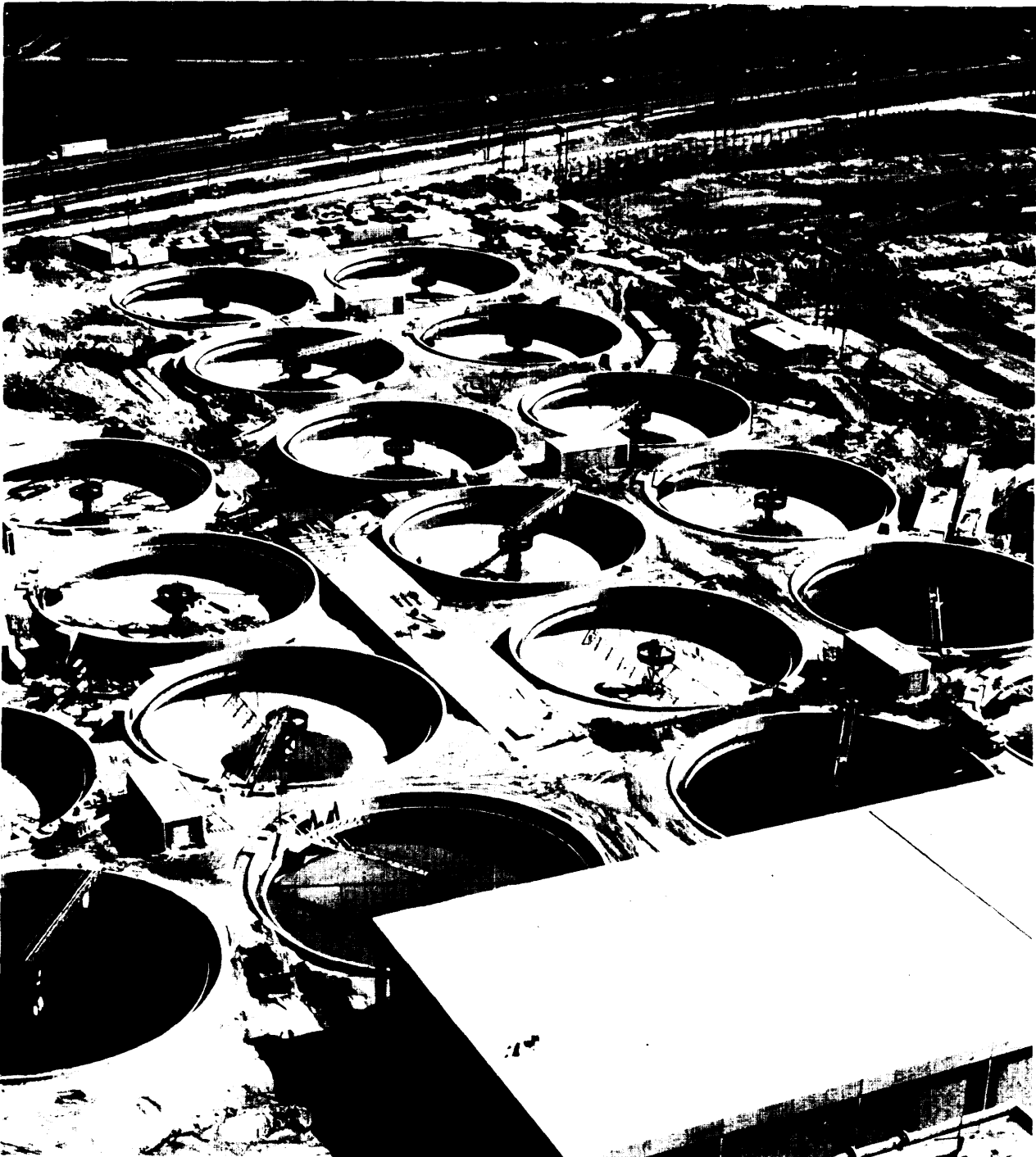
Sewage treatment plant, Blue Plains, Maryland
