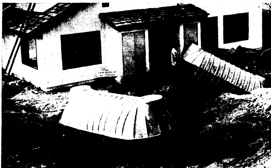
Figure XI-4.— Installation of Fiberglass Underground Tanks
