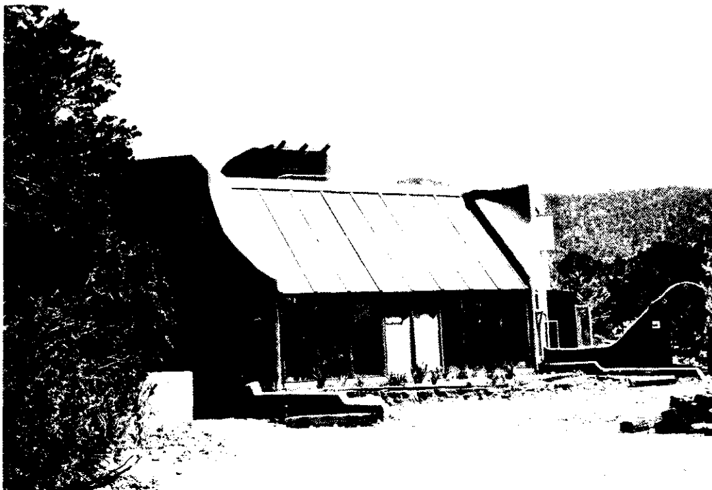
Figure 52.—The Balcomb Home Near Sante Fe, N. Mex., Combines the Use of a Greenhouse With a Rock Storage Bed to Provide 95 Percent of Its Heating Needs
