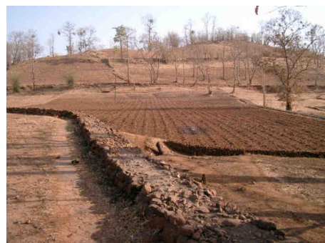
Figure 3.10: A well-made bund
