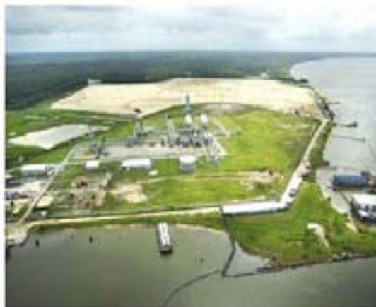
Aerial photo of the GTL plant at Escravos, Nigeria. Photo courtesy of Sasol Chevron
