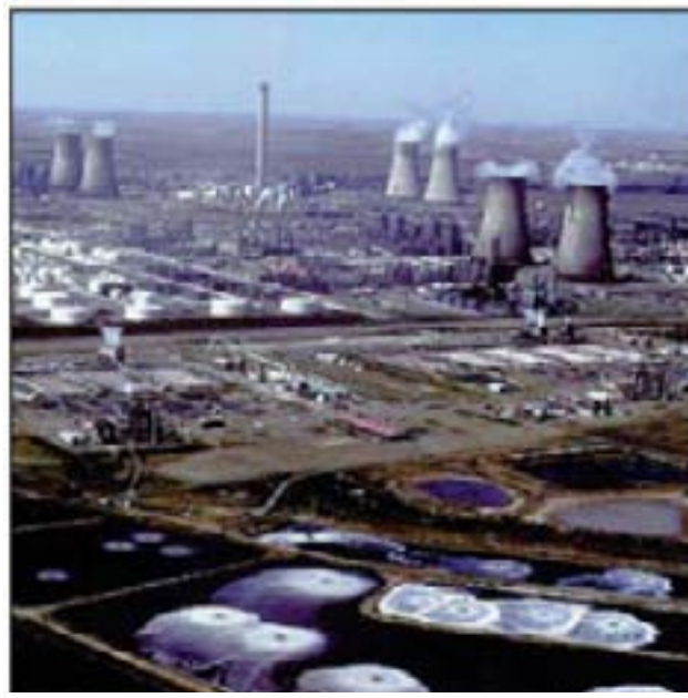
Source: Sasol CTL plant in South Africa, Cleaner Coal Technology Program. London, UK
