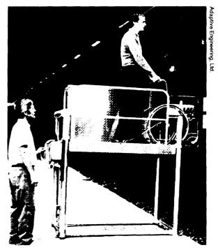
This station-based lift, while designed for use on rail systems, may be adapted for OTRBs.
