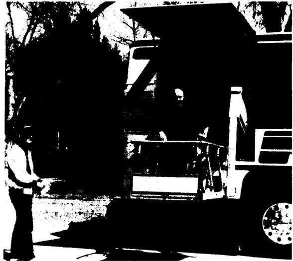
*A man in a wheelchair uses one of several available OTRB vehicle-based lifts.*
