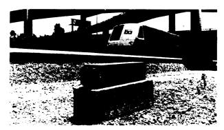
FIGURE 15.—Wayside Equipment Case (contains multiplex equipment for transmittin, information between trains and station control rooms)
