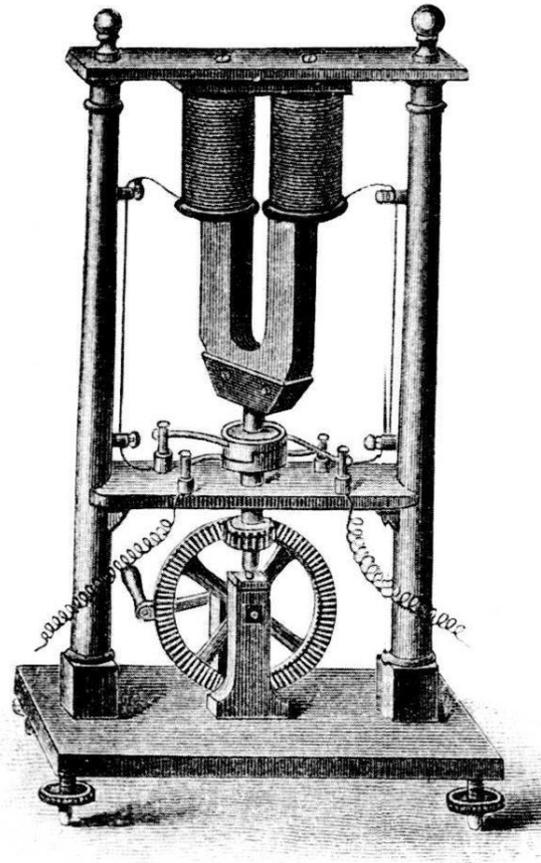
*Hippolyte Pixii's dynamo. The commutator is located on the shaft below the spinning magnet.*
