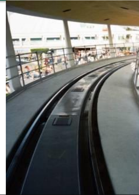
Active element of LIM in guideway
