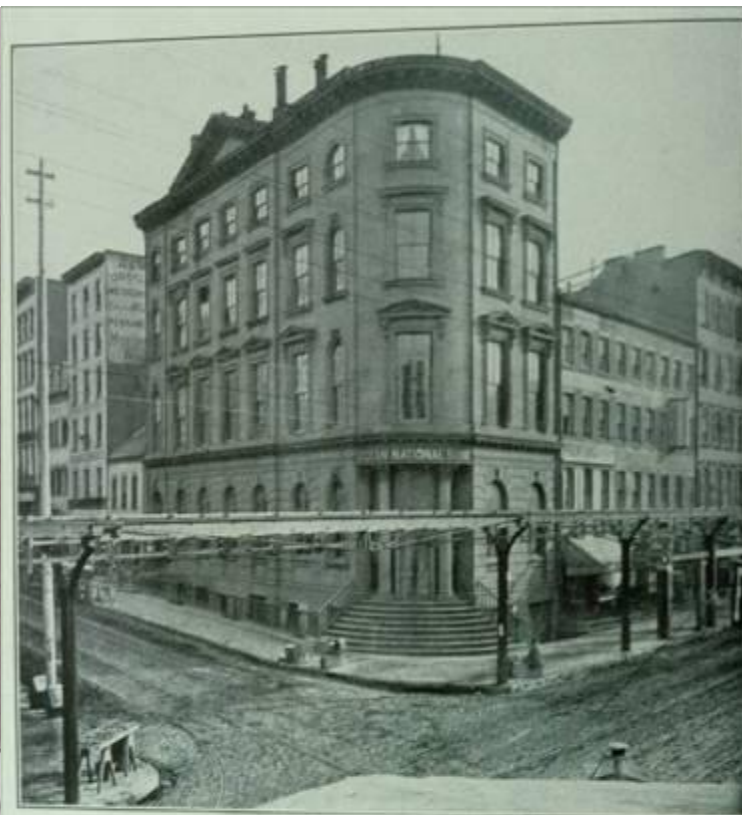
GREENWICH STREET, LOOKING SOUTHEAST FROM THE CORNER OF FULTON STREET, 1869 Showing the first elevated railroad, erected 1868-69 on the easterly curb line of Greenwich Street in front of the Ocean National Bank, and operated by cable.
