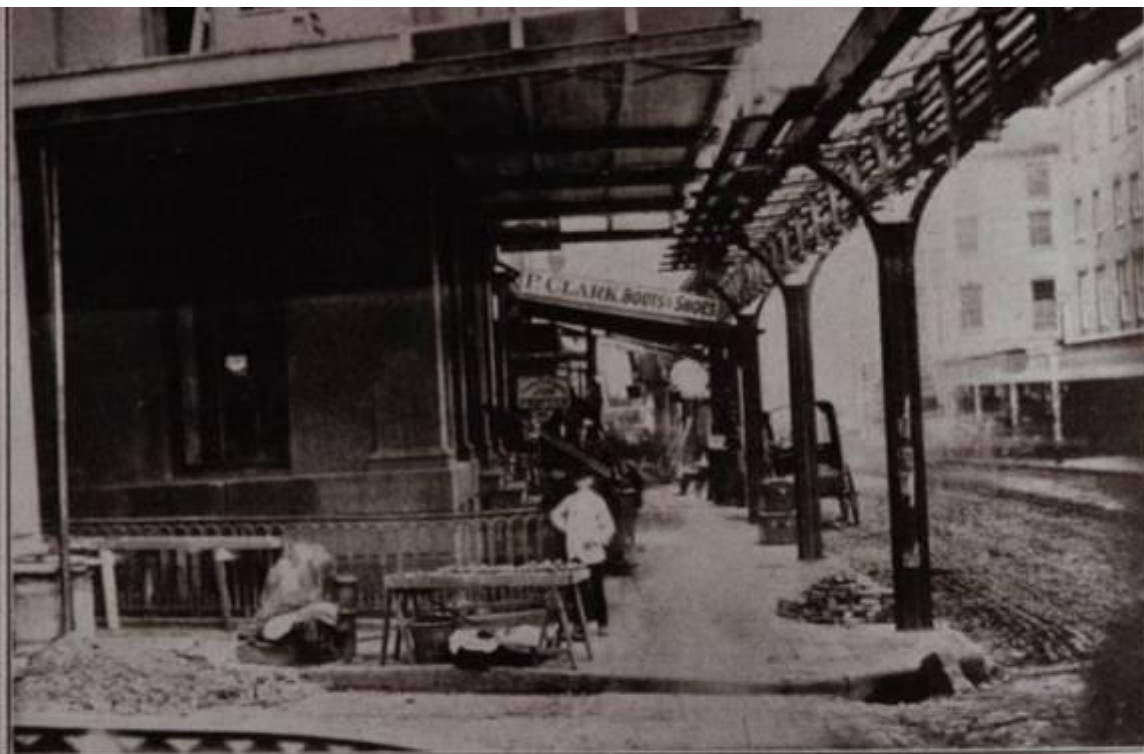
GREENWICH STREET LOOKING SOUTHEAST FROM DEY STREET, 1868-69 Showing the elevated structure on the east curb line of Greenwich Street, built in 1868-69, cable used for train operation, showing the first south station at Dey and Greenwich Streets in course of construction.
