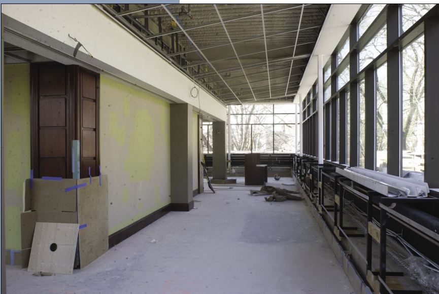
One wing of the new third-floor study and seminar room area
