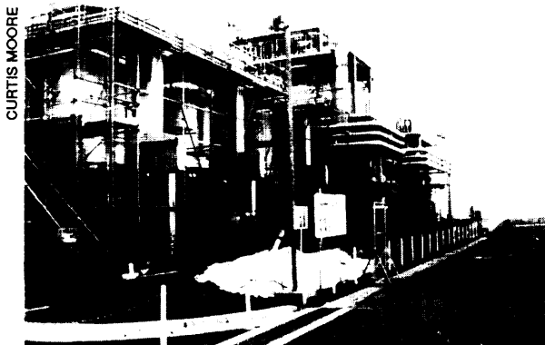
Tokyo Electric Power Company's 11 megawatt phosphoric acid fuel cell is the largest fuel cell installation in the world. Most of Japan's environmental R&D concentrates on improving energy technologies.
