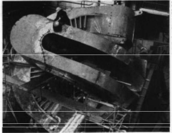
End magnets for the Mirror Fusion Test Facility (MFTF-B)
