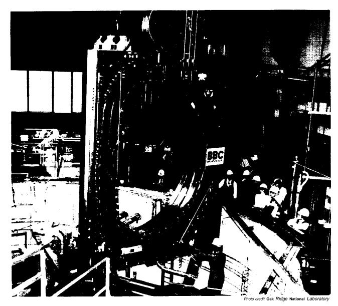
The Swiss superconducting magnet coil being installed in the International Fusion Superconducting Magnet Test Facility (Large Coil Task) at Oak Ridge National Laboratory.
