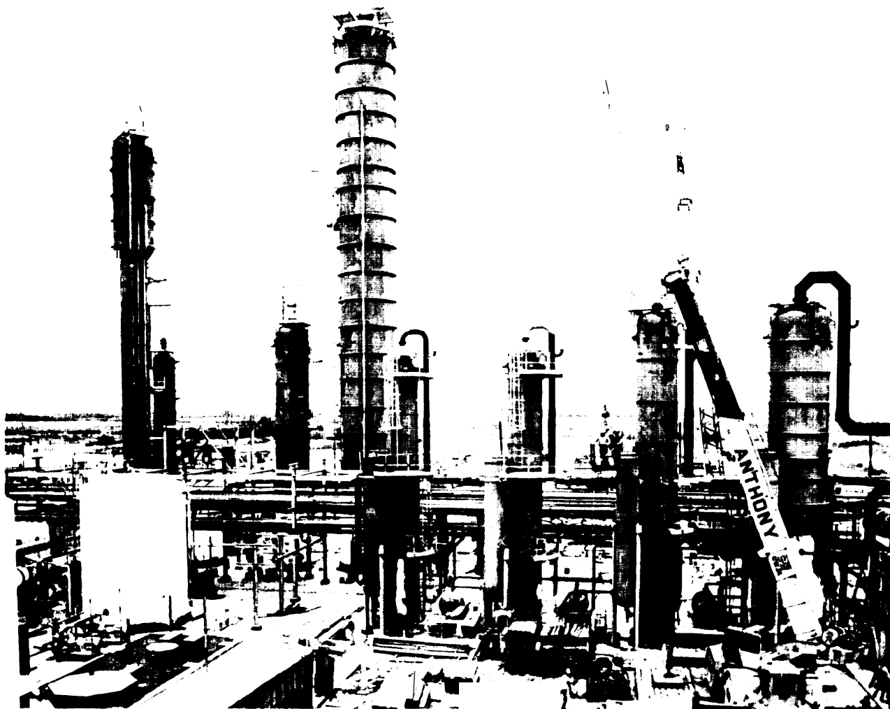
Photo credit: PPG Industries, Inc
