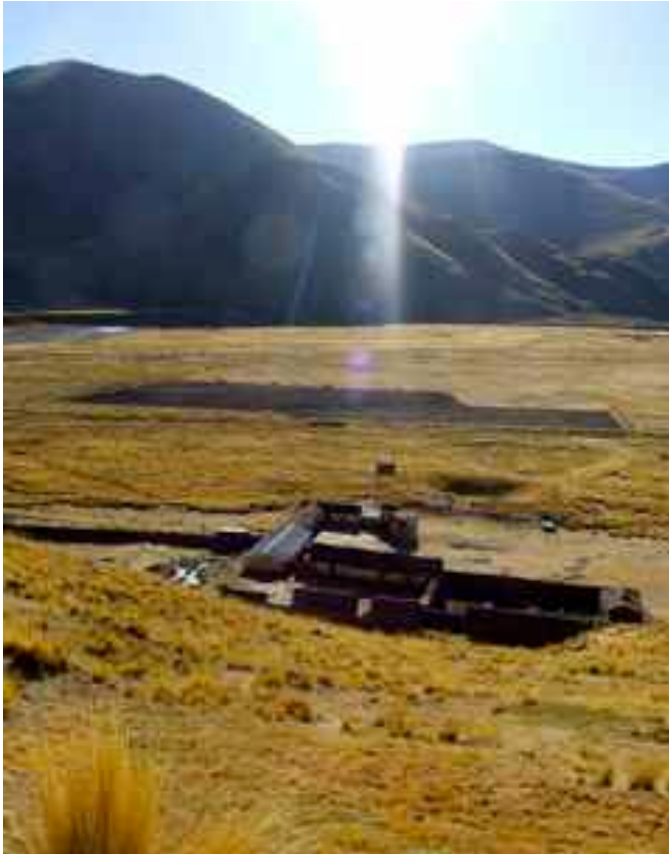
Overlooking Diego Tapara's communal buildings and masa on an early morning in July.
